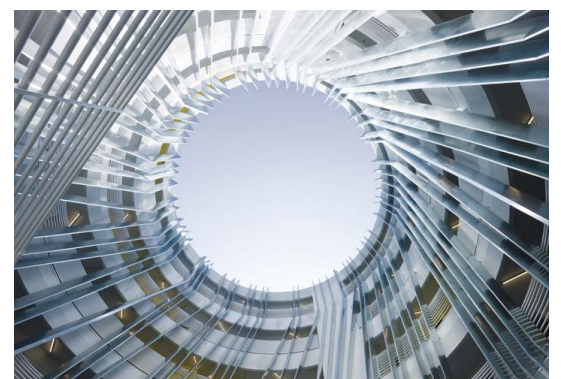
New Carver Apartments Courtyard © Iwan Baan
